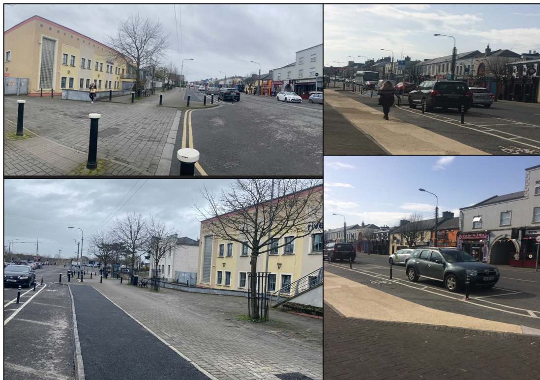
Figure 6. AECOM Site photos of R778 Main Street
