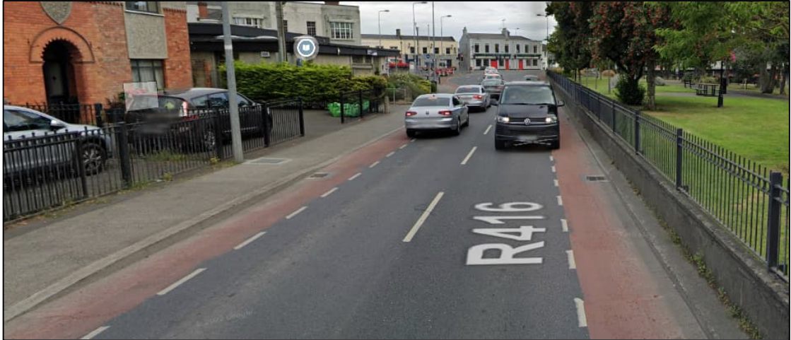
Figure 7. Existing Cycle Facilities Athgarvan Road
